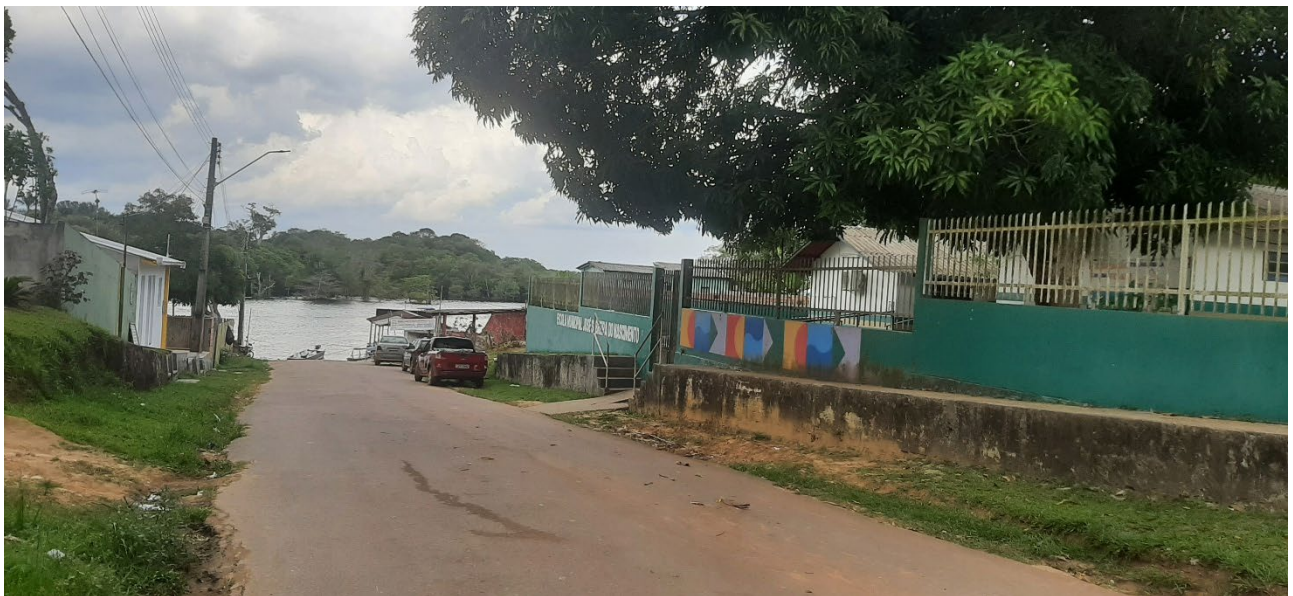
Figure 4 | Photography of José Sobreira do Nascimento Municipal School, in the Nossa Senhora de Fátima Community, Manaus-AM.
